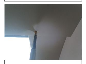
**STEP 3)** Using 2 x screws 3.5x25 (Part No: **1430058**) fix the CPL to the blind cap.
