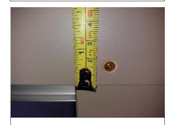
**STEP 4)** Ensure each of the screw heads are flush to the CPL.
