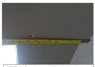
**STEP 1)** Start by pre-drilling holes through the CPL on both sides at 85mm from the side edge and 15mm up from the bottom edge.
